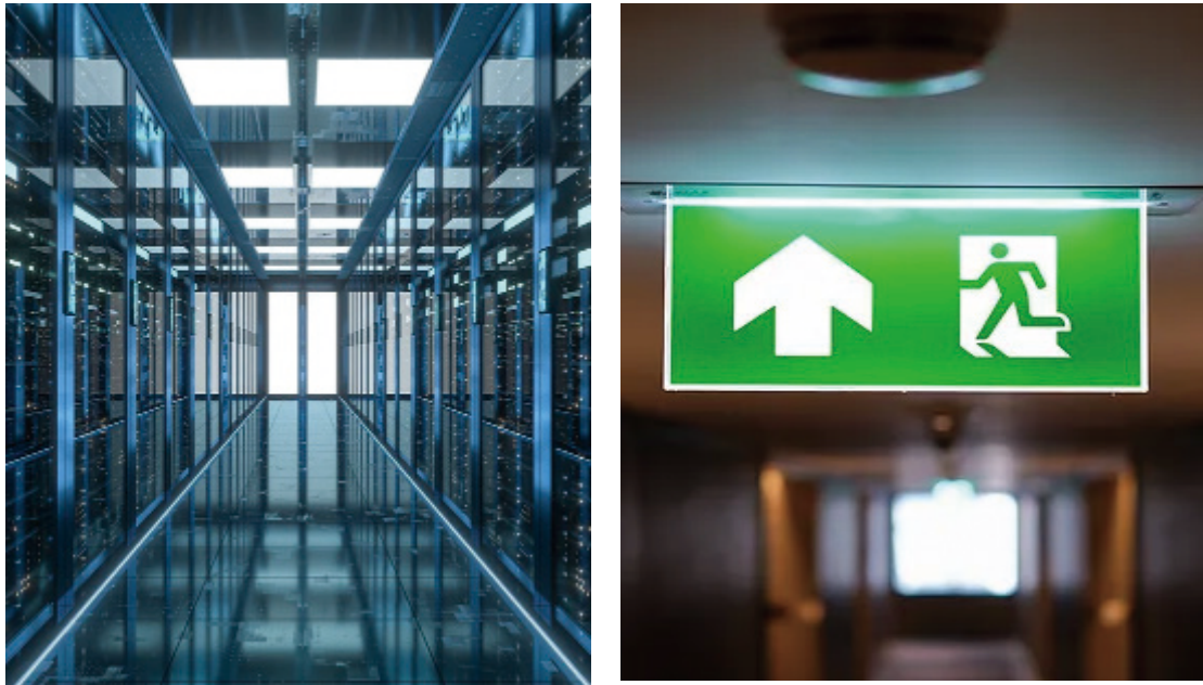
Figure 6. Uninterrupted Power Supply and Emergency lighting
